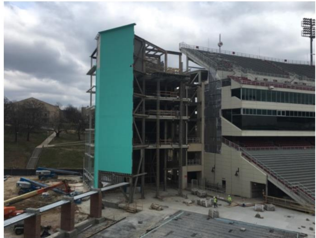
44 - 11 NE Stair Tower
