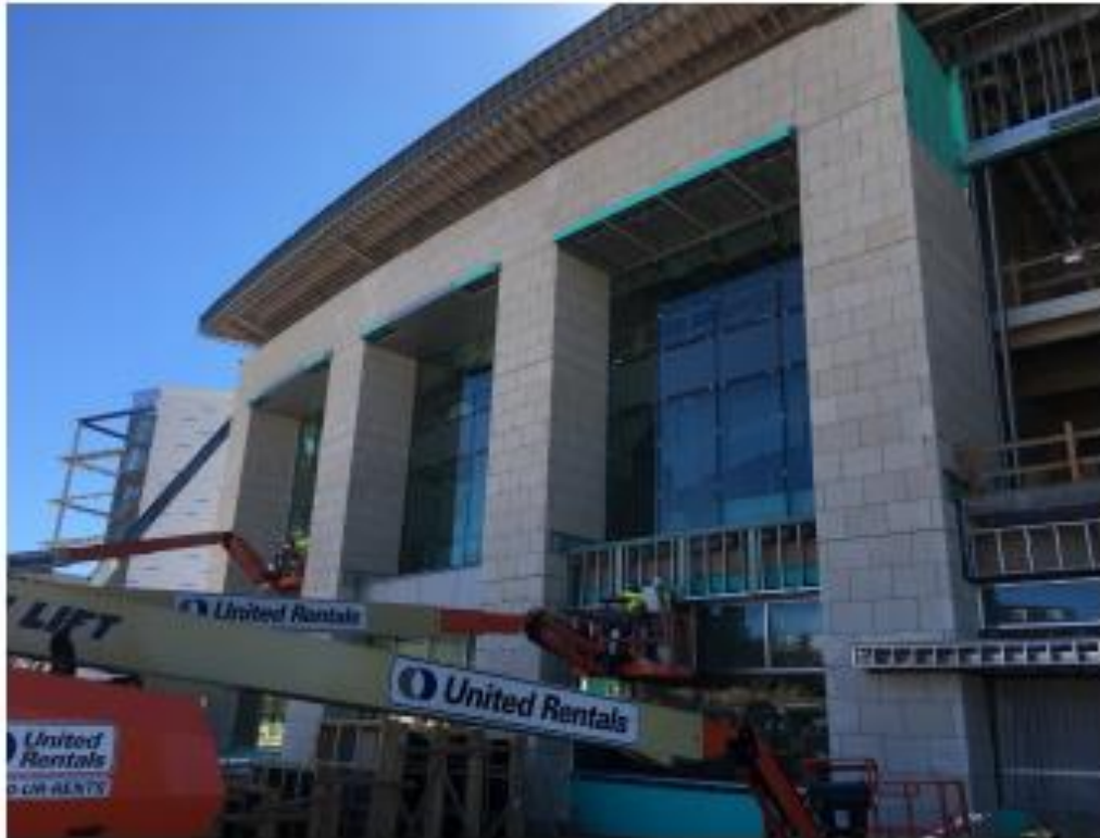
43 - 11 North Elevation Masonry, Glazing and Metal Panel progress
