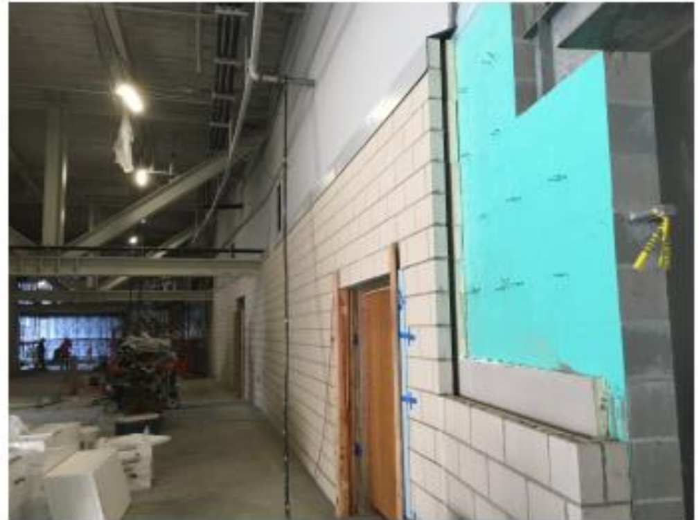
43 - 06 Masonry & EFIS Progress at Level 02 Concourse
