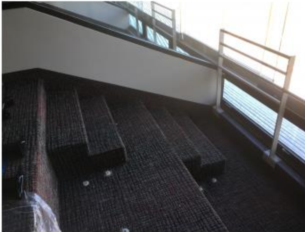
43 - 03 Renovation Progress in West Lower Suites
